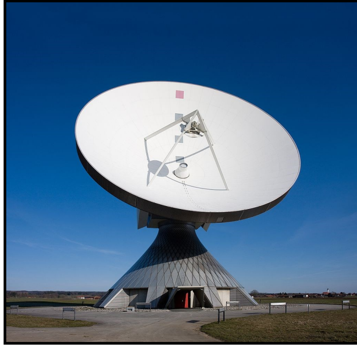
Figure 2.9 The photography of a large parabolic satellite communications antenna at Erdfunkstelle Raisting in germany. [45]
