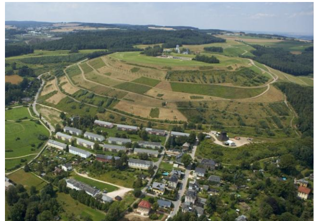
Figure 1. Waste rock dump 38neu of uranium mining in Bad Schlema, Wismut GmbH, Germany. Note proximity of housing developments near the dump toe
