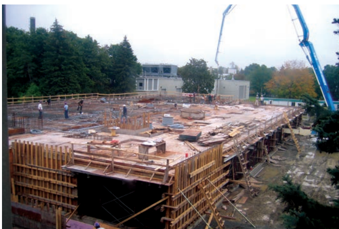
Building 18-PRF (research and training centre) under construction in 2006 © INRS Archives Photographer: Sylvain Millot
