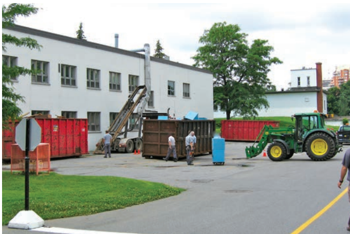
Building 12 under renovation (2006) © INRS Archives Photographer: Pierre Payment
