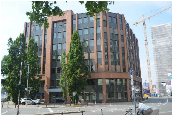
Figure 11: Edifice Ubisoft Düsseldorf, Adlerstraße (until August 2019)
