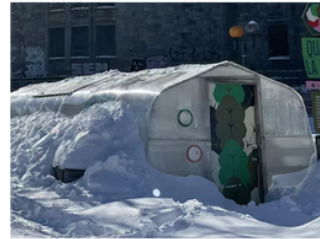
Single polyethylene (PEs) greenhouse, unheated. South Central, Montreal
