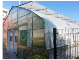
Double polyethylene (PEd) greenhouse, active ventilation and gas heating. South Central, Montreal
