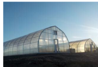
Polycarbonate (PC) greenhouse, active ventilation, storage system and unheated. Kuujuaq, Nunavik
