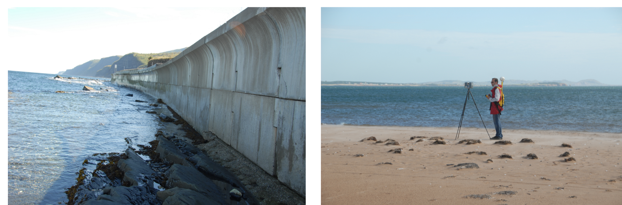
Seawall protecting the road Beach surveying, Magdalen 132, Gaspé Peninsula, Islands, Quebec. Quebec.
