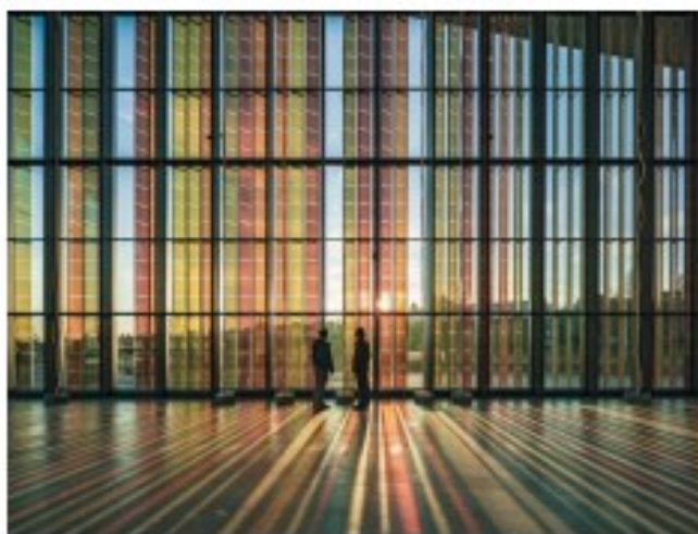
Figure 1-7 DSSC façade at the SwissTech convention center at École Polytechnique fédérale de Lausanne (30)
