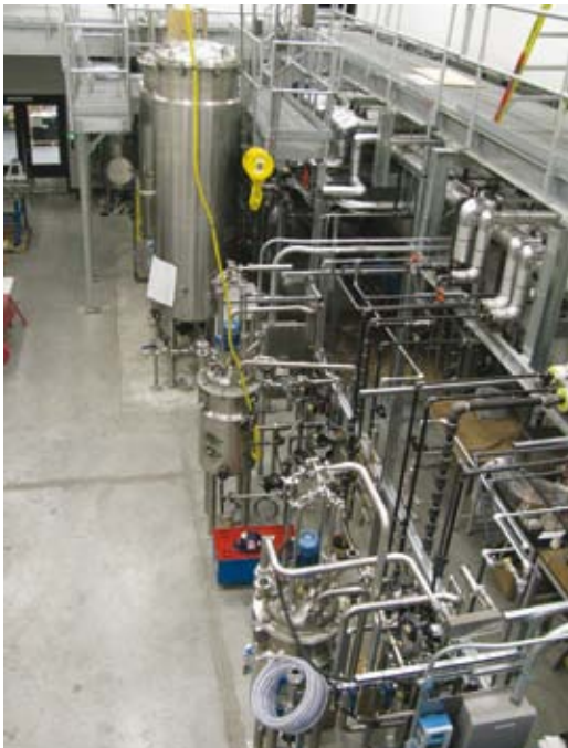
Fermenters for decontamination work
