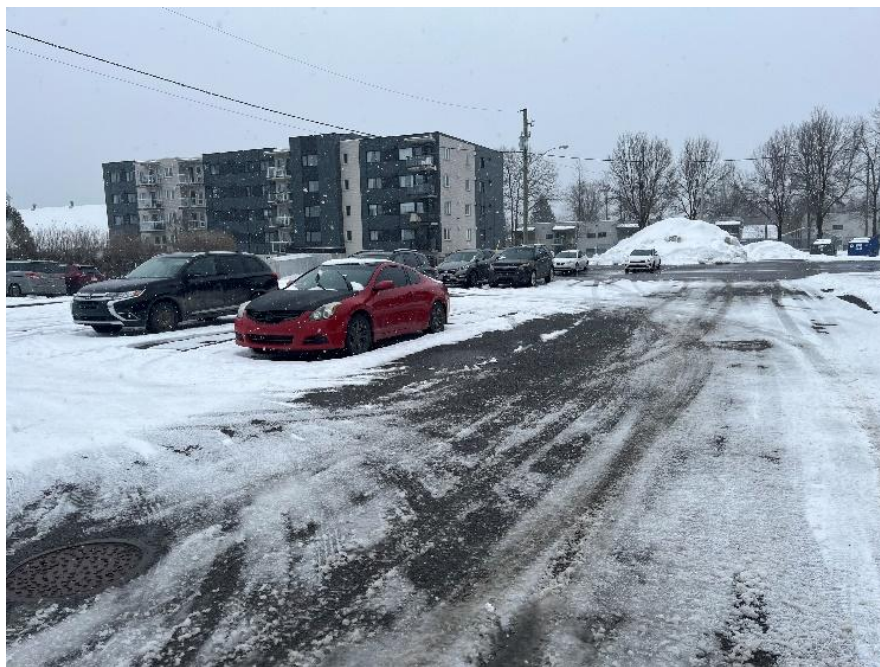
Figure 4-4 Sediment accumulation on the main driving lanes of the porous parking lot area
