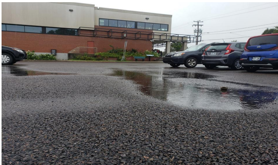
Figure 4-2 Surface water pooling on permeable asphalt (photographed on September 18, 2023)
