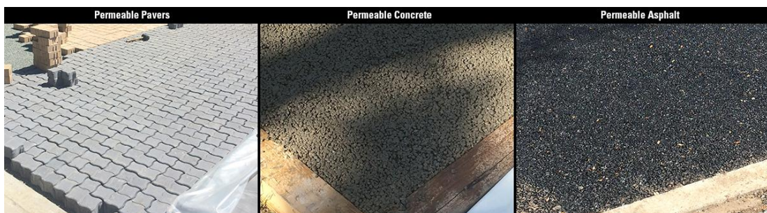
Figure 2-1 Different types of permeable pavements ( Selbig & Buer, 2018)
