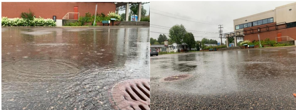
Figure 4-3 Pooling of water on the permeable asphalt surface (images captured on June 7 and 23, 2024, respectively)
