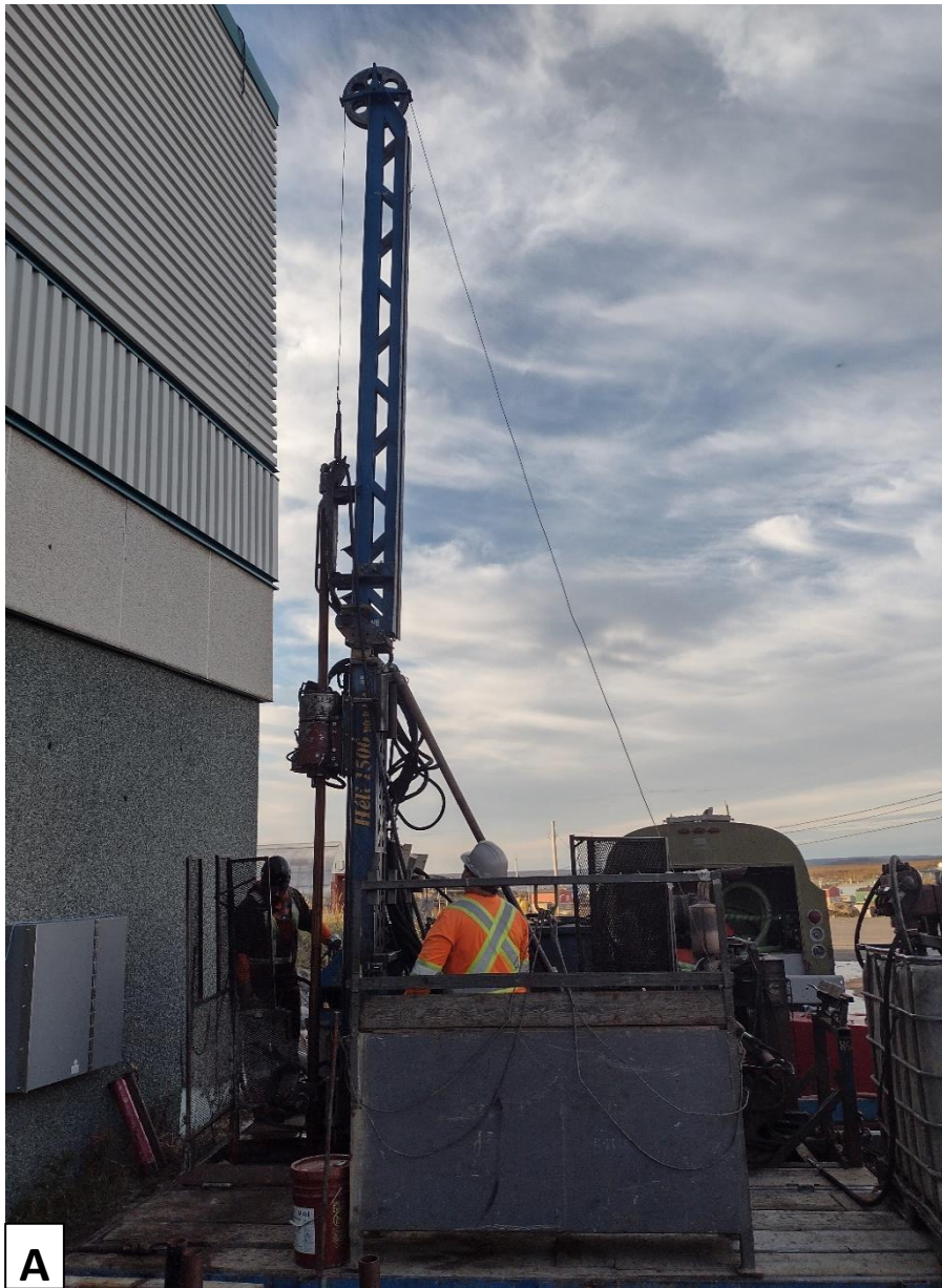
Figure 4 – The vertical diamond drill hole next to the mechanical room of the Forum building in Kuujjuaq. B – Removal of the sand plug that was left due to the failure of the first ground heat exchanger installation attempt in 2021.
