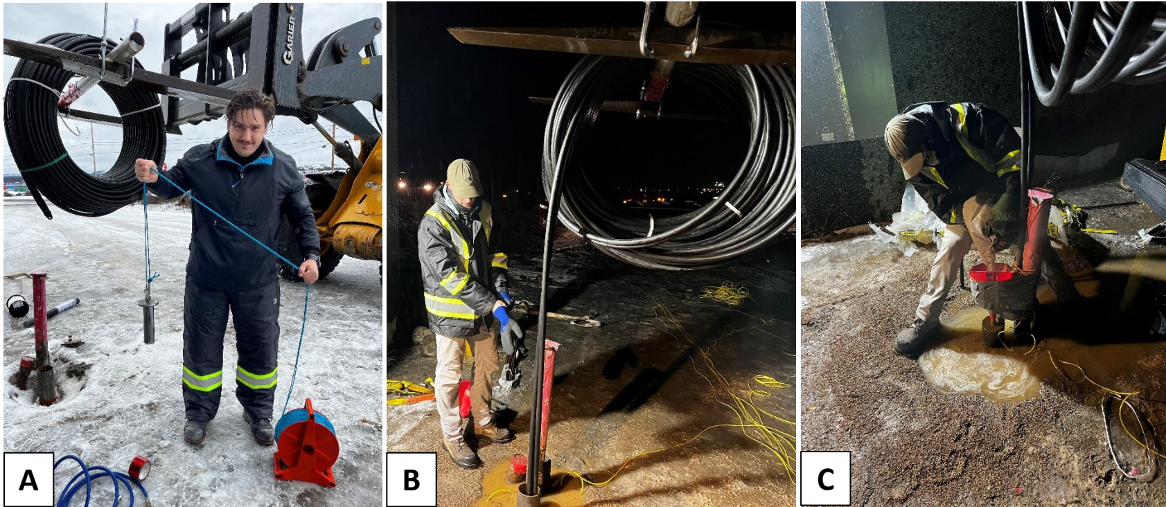
Figure 15– Vertical ground heat exchanger installation. A-A plug was inserted at the bottom of the NQ hole prior to B-the U-pipe installation, which occupies the 122 m depth of the upper part of the well , C-then the borehole was backfilled with coarse sand. Credits Induktion Géothermie.
