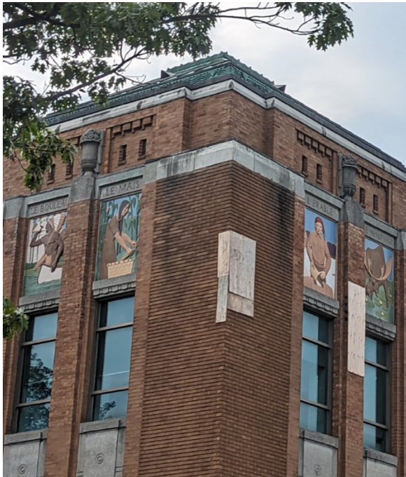
Figure 3.10 : Murals on the main building of the Botanical Garden of Montreal
