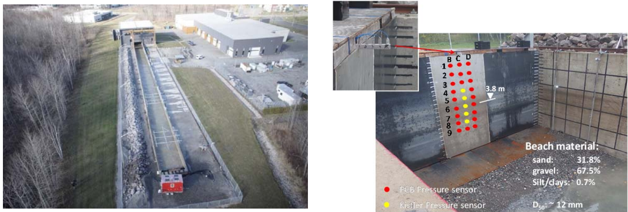
Figure 2. Experimental set-up (wall without parapets).
