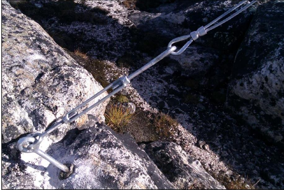
Figure 28 : Guy-wire with jaw/eye turnbuckles
