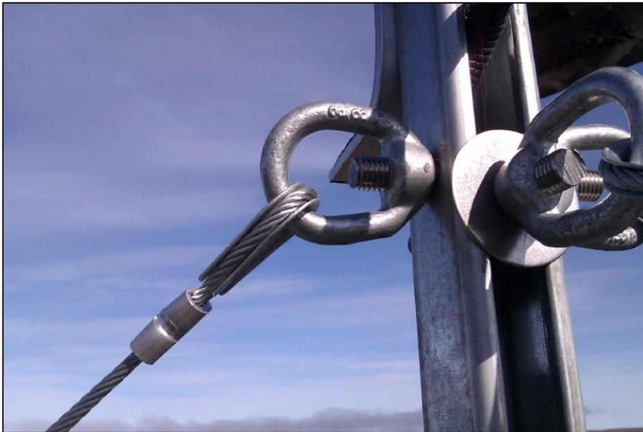
Figure 29 : Guy-wires fixed with eye nuts and threaded rod
