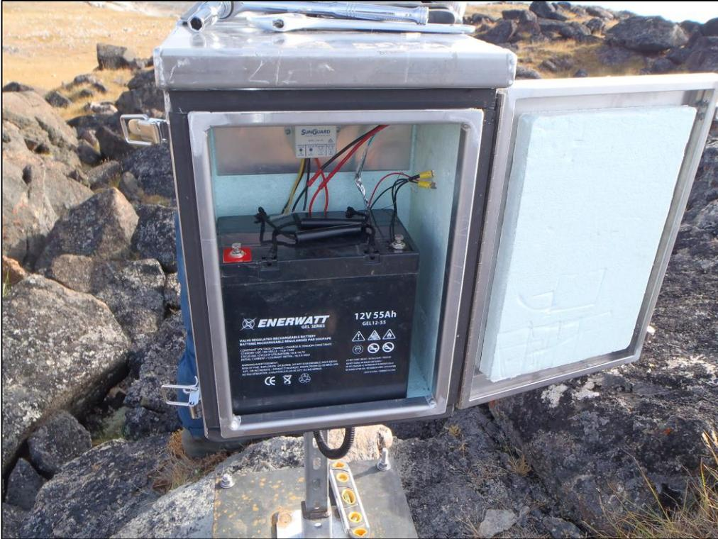
Figure 31 : Solar charge controller and 12V battery
