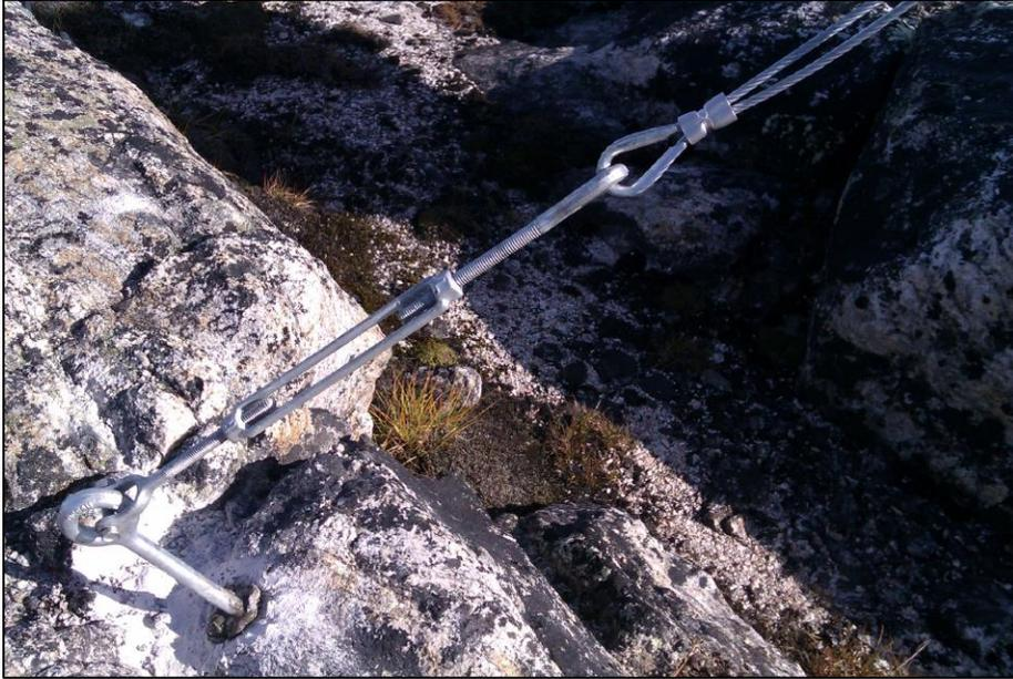
Figure 28 : Guy-wire with jaw/eye turnbuckles
