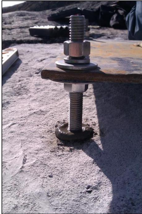
**Figure 27 : The structure is fixed with threaded rod and leveled with nuts and washers**
