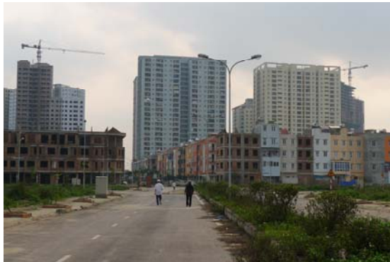
Figure 1: Van Khe, a redevelopment under construction at the periphery of Hanoi, April 2013. Credit: Danielle Labbé
