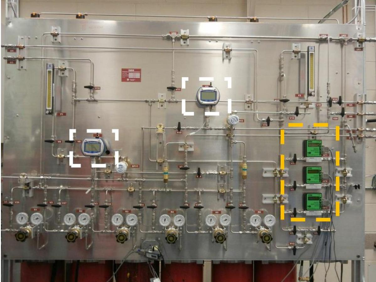
**Figure 3. 6** – Gas panel evidencing the mass flow meters (yellow dotted square on the right) and the pressure gauges (white dotted squares).
