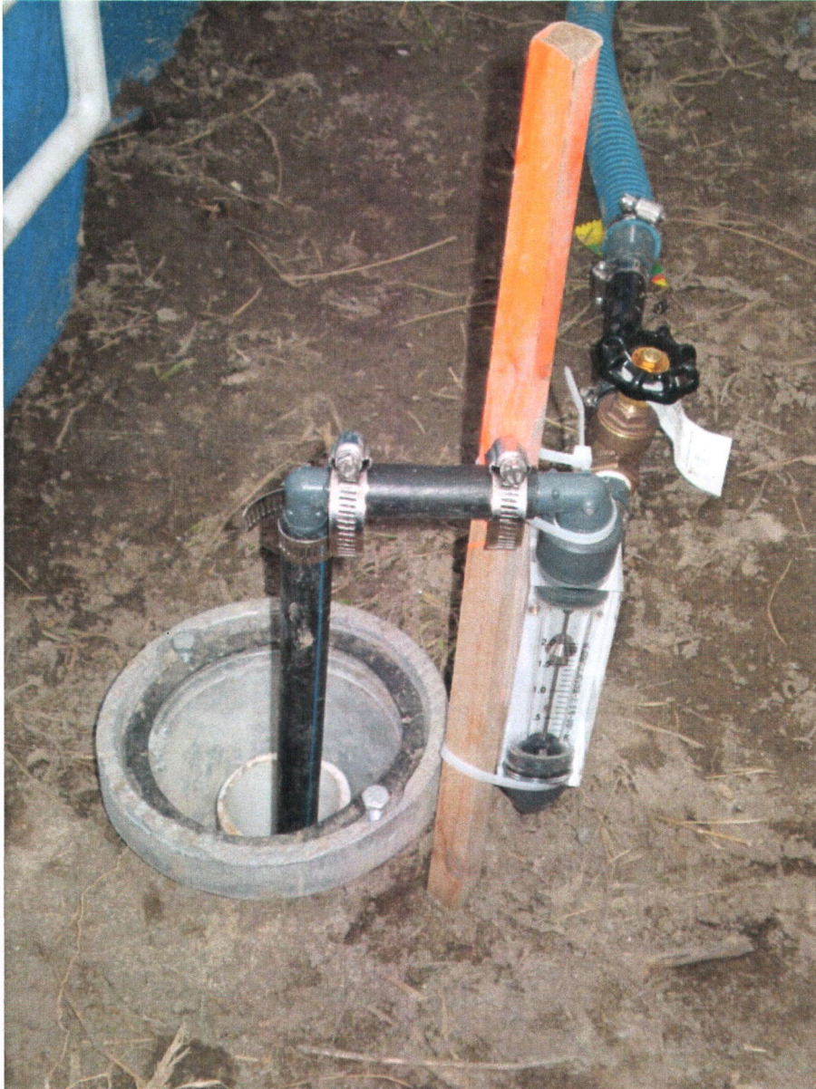
Figure 3.5. Gate valve followed by flowmeter on the injection line
