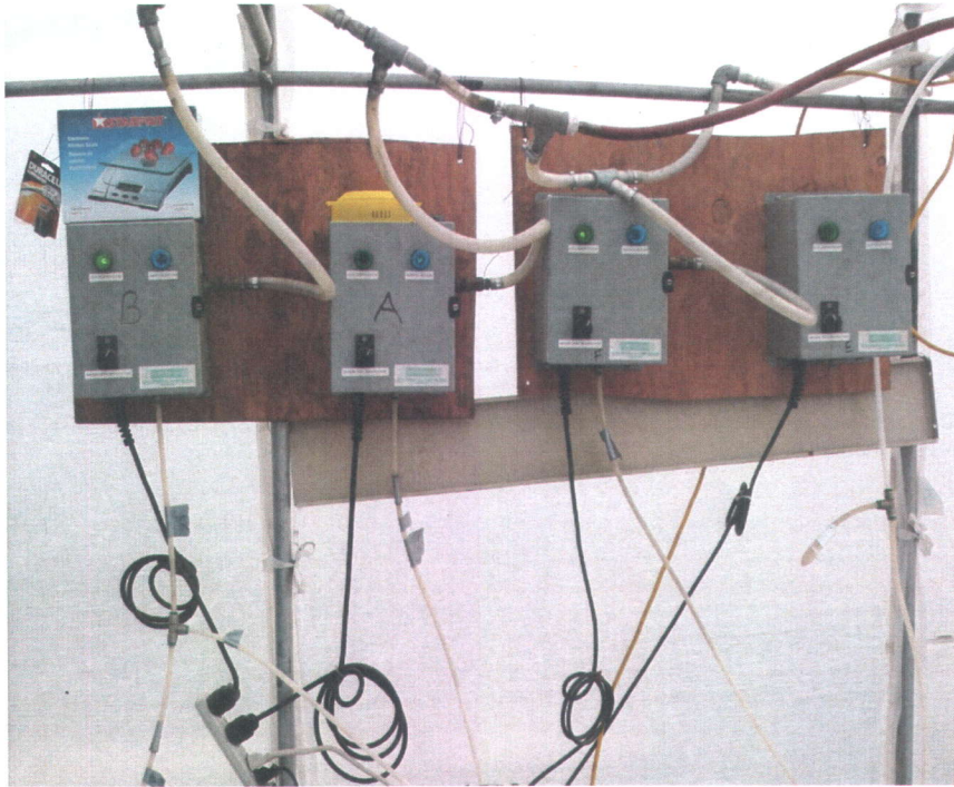
Figure 3.6. Control panels for bladder pumps
