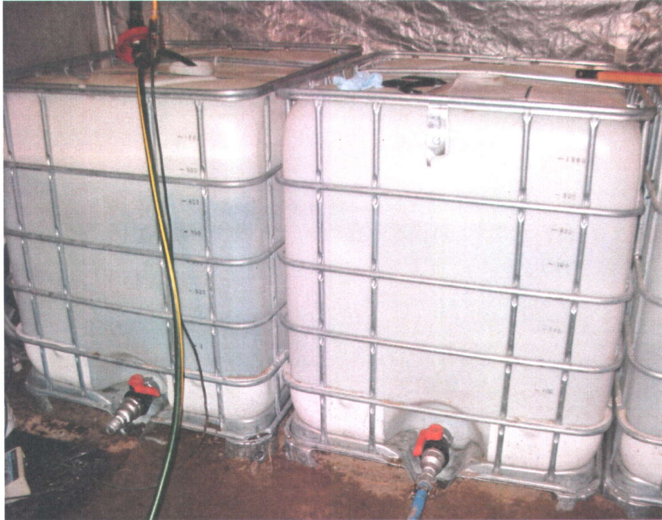
Figure 3.3. 1 m 3 tote tank containing injection solutions
