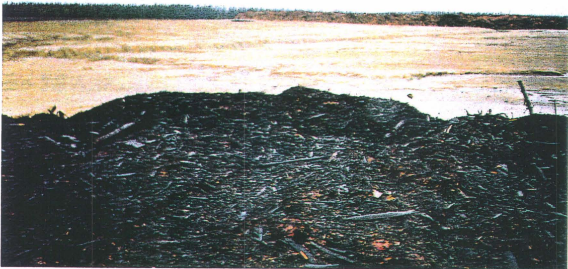
Photo 2: Photo taken from the top of the organic cover showing the mine tailings with the inner edge of the organic cover in the distance (October, 1996).
