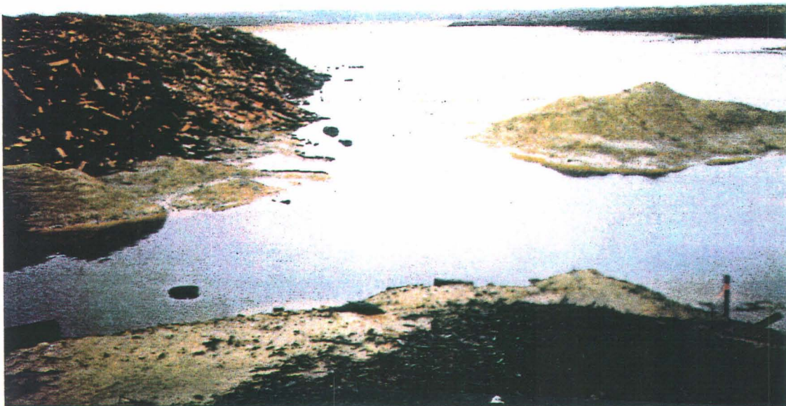
Photo 1: Mine Tailings impoundment with a retention dike in the foreground and the limit of the organic cover in the distance (October, 1996).
