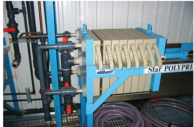
Filter press for sludge dewatering
