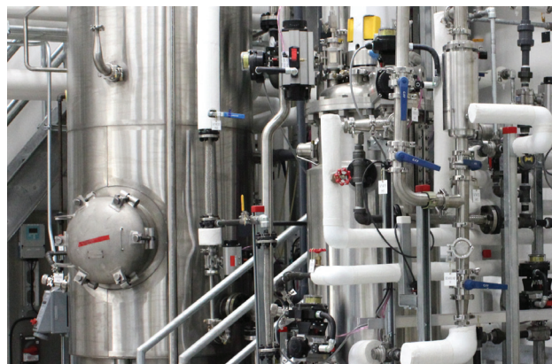
| 2000-litre capacity hydrolyzer
