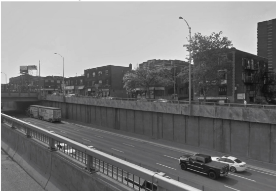
c. Road in cutting
