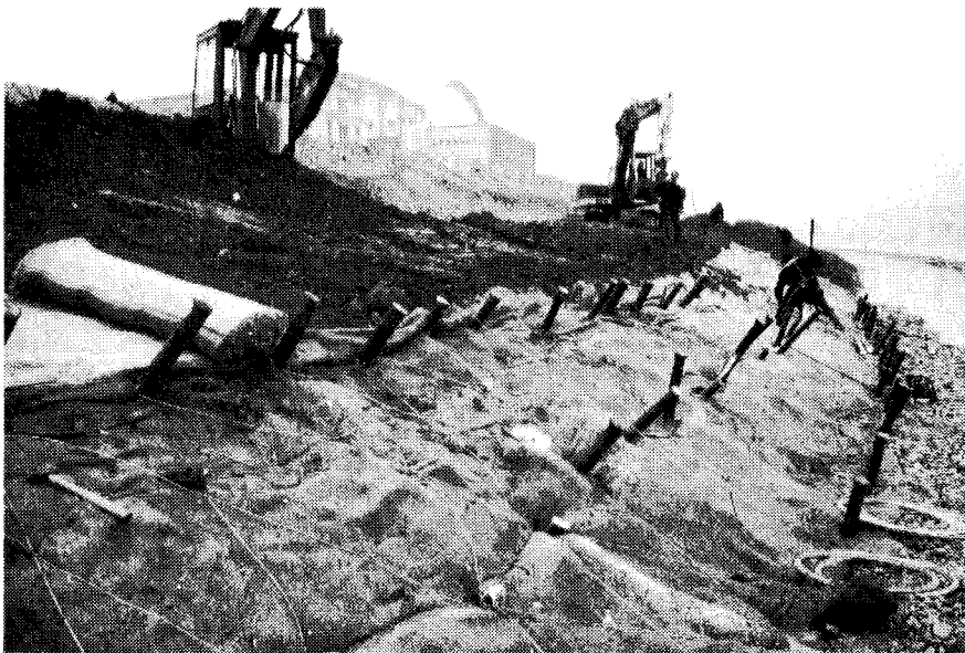
Figure 8.b: Layering of branches of 5 species of willow, covered by a putrescible geotextile and fixed by willow stakes. January 24, 1994 (Photo : B. Lachat)
