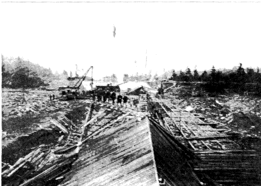
Figure 4. Photographs of the Donnacona dam in 1913. (Domtar 1989)
