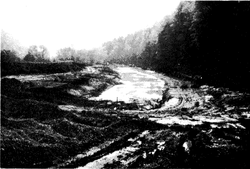
Figure 7.a: Digging the new river bed. June 1, 1984 (Photo : B. Lachat)
