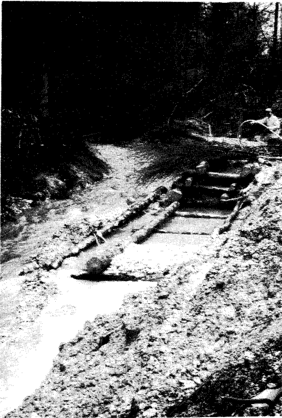
Figure 6.b: Installation of the crib frame for earth, cuttings and plants. November 26, 1992 (Photo : P.A. Frossard)
