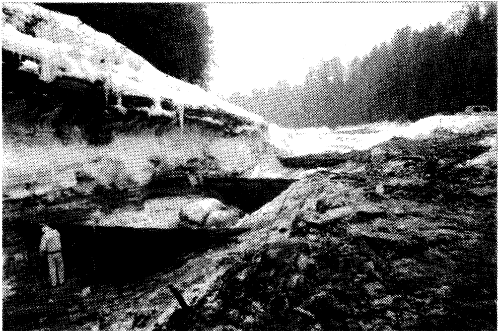
Figure 15. The Déry gorges during pre-dam construction.
