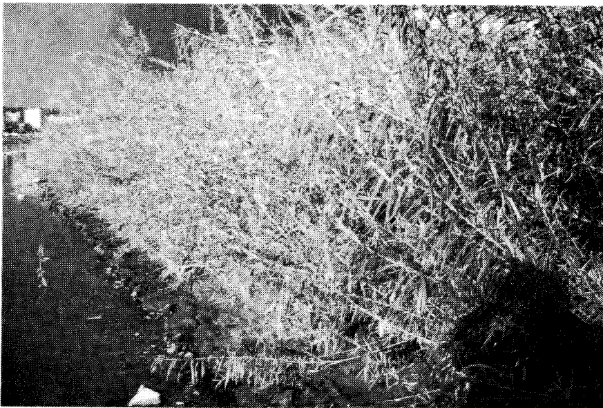
Figure 8.f: A few months later, vegetation has grown to form water- resistant bushes. One species of willow (saule des vanniers) is dominant. Even on large streams, bioengineering techniques can be applied. September 8, 1994 (Photo : B. Lachat)
