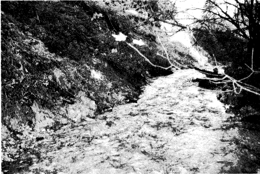
Figure 6.a: The bank prior to intervention. Erosion and landslides were threatening a road on the bank crest. October 29, 1992. (Photo : B. Lachat)
