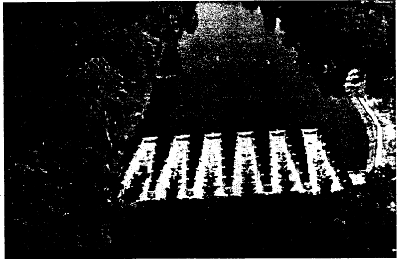
Figure 4. South Holston Labyrinth Weir
