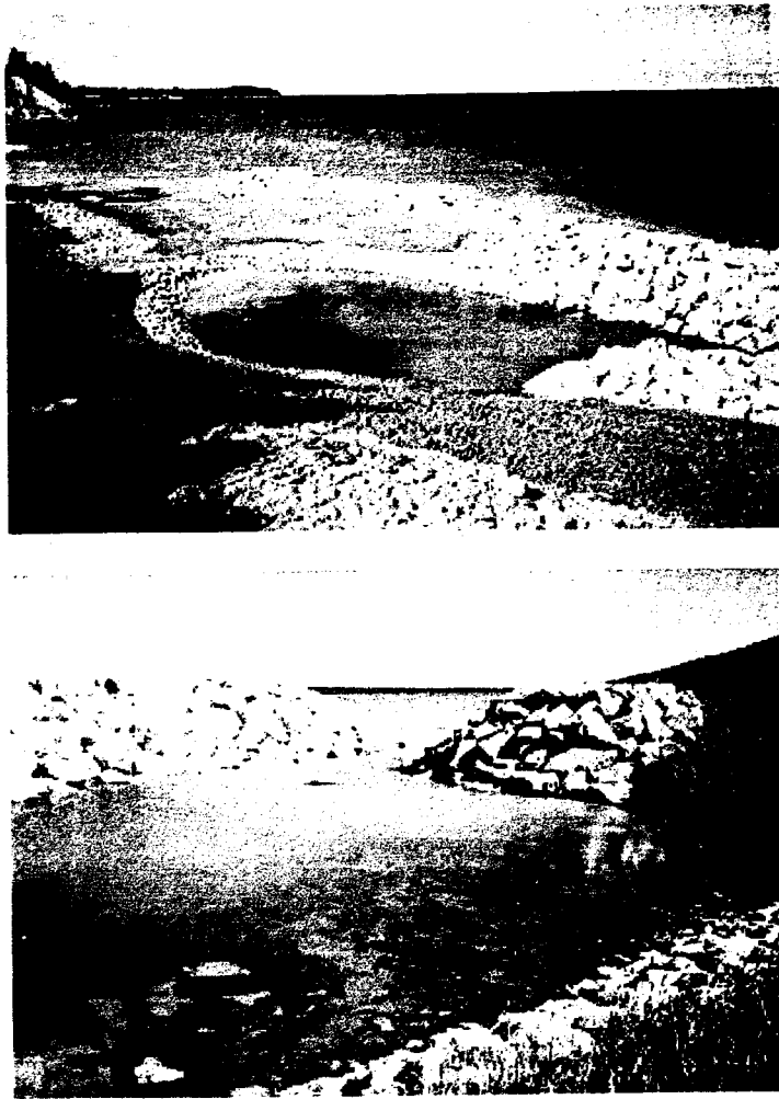
FIGURE 6 BENDER PARK LOW WAVE ENERGY CONSTRUCTED LAGOON
