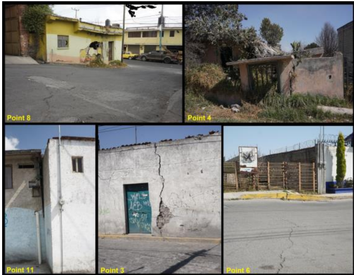
Figure 11: Examples of ground fractures observed in the field while surveying the areas identified by PSI. The locations visited are all marked on Fig. 10. In some locations, obvious linear ground fractures are found (e.g., points 8, 4, and 6), while in others, only discontinuous subsidence effects can be observed (e.g., points 11 and 3). The latter can be interpreted as secondary effects of structural damage suggesting the possible occurrence of differential subsidence and ground ruptures.
