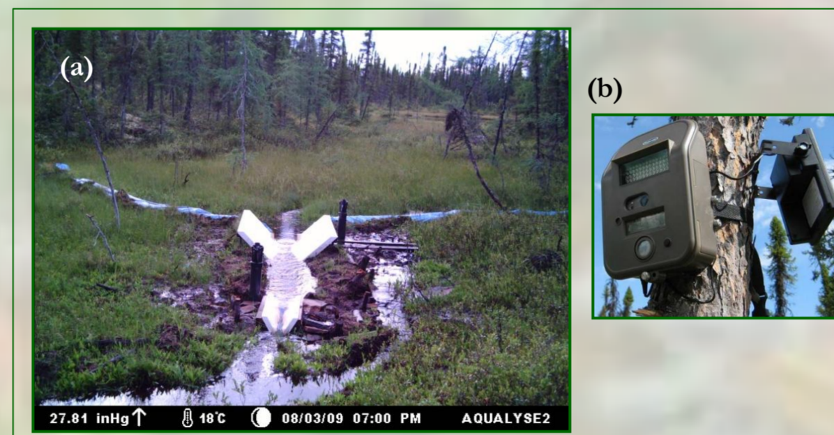
Figure 4. (a) Trapezoidal channels at the outlet of the watershed and (b) the camera, that automatically take one picture every hour, installed in front of the channels
