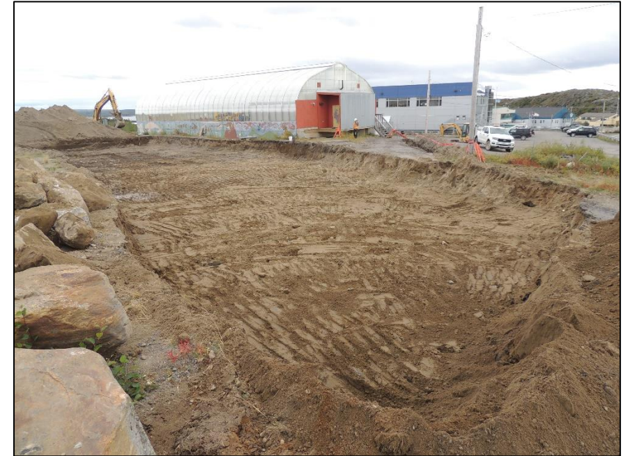
Figure 14 – Northern part of the excavation.
