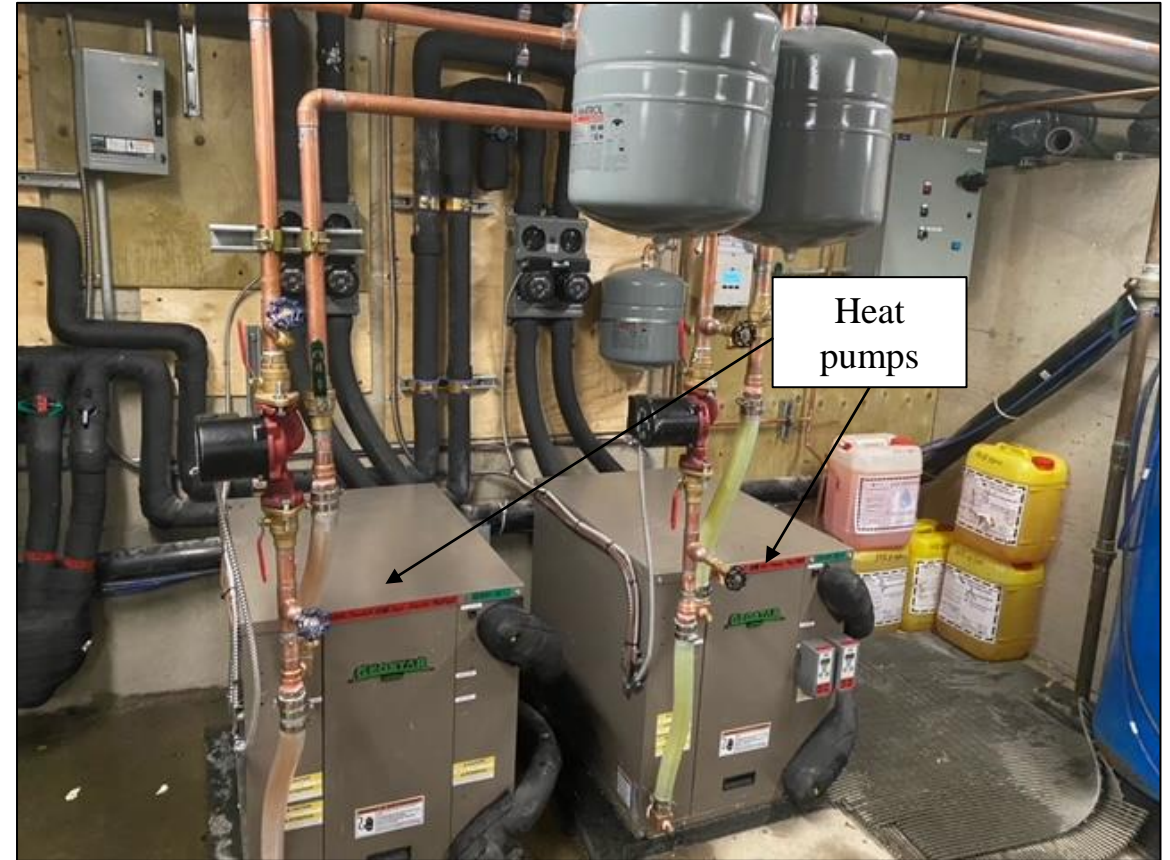
Figure 12 – 16 HDPE pipes (IN and OUT of 8 loops) entering the mechanical room and connected to the two heat pumps (November 2020, Credits Pierre Vallerand, Induktion Géothermie)
