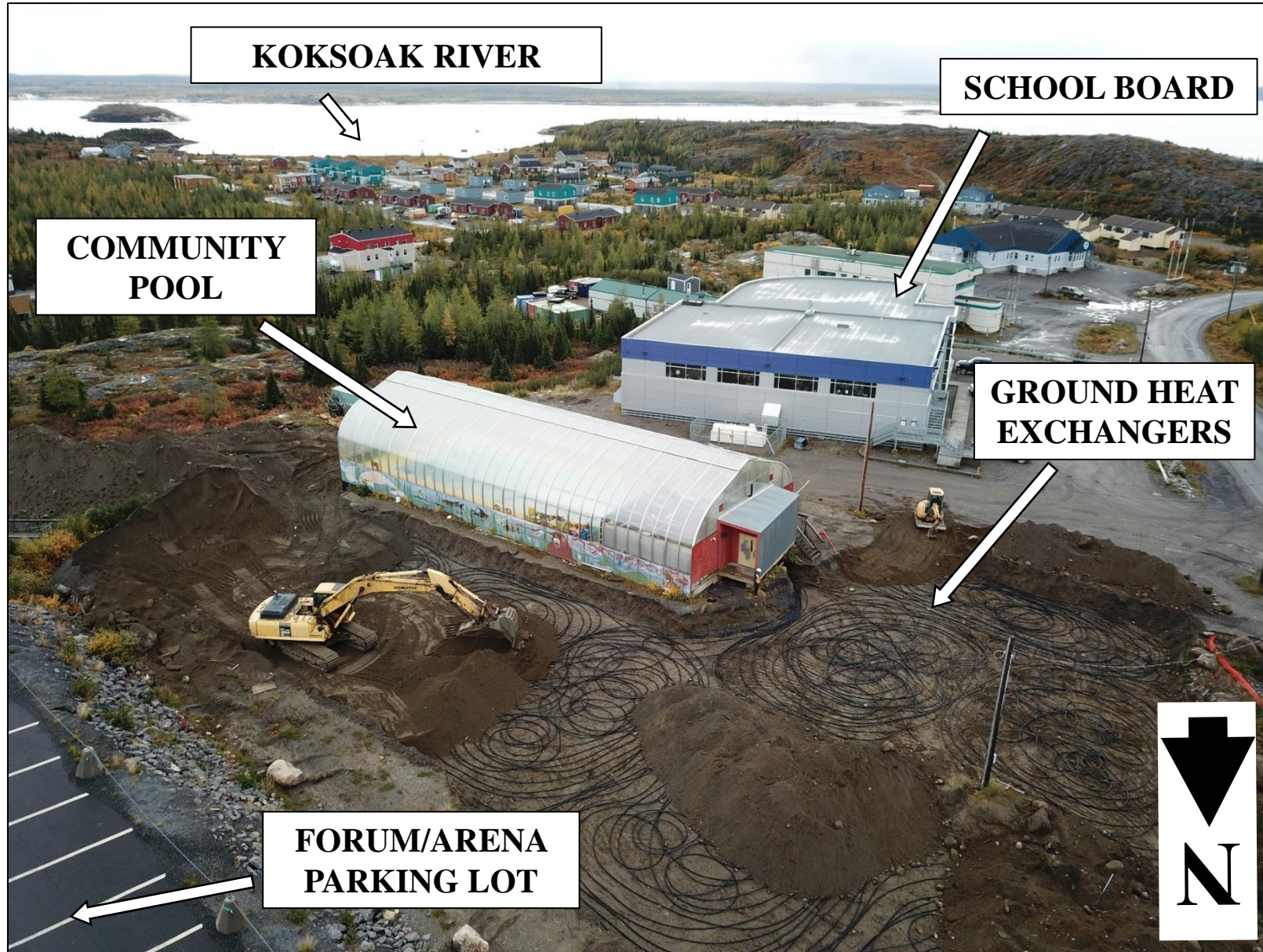
Figure 6 – Aerial view of the ground-source heat pump system at the Pool in Kuujuaq (September 2020, Credits Jason Aitchison, Kuujjuamiut Inc.).
